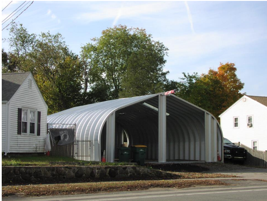
Example of inappropriate accessory building located in a residential district on Dean Street near Tamworth Road.
